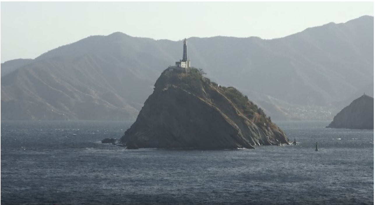
Lighthouse topped island at the entrance to Santa Marta harbour
