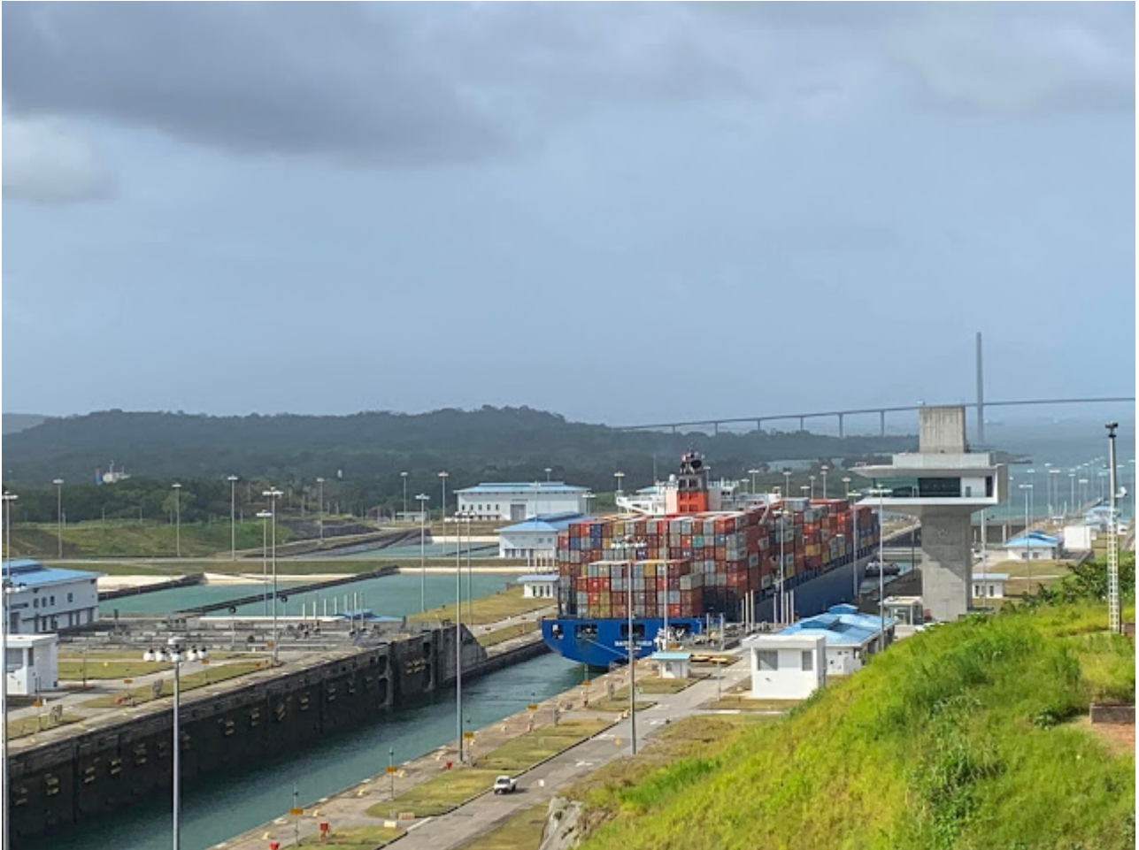
One of the locks on the Panama Canal
