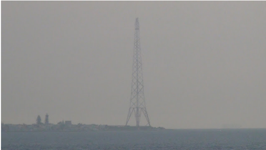
800ft high power pylon
